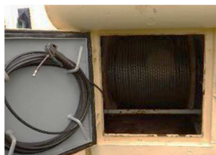
Figure 4 - Opened access panel of winch room
