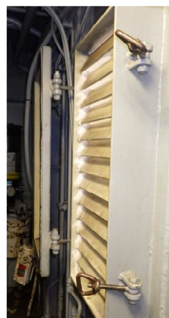
Figure 11- Closing panel for ventilation opening inside the winch room
