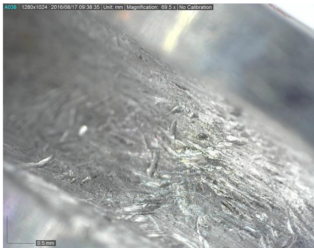
Figure 5: pulley groove damage
