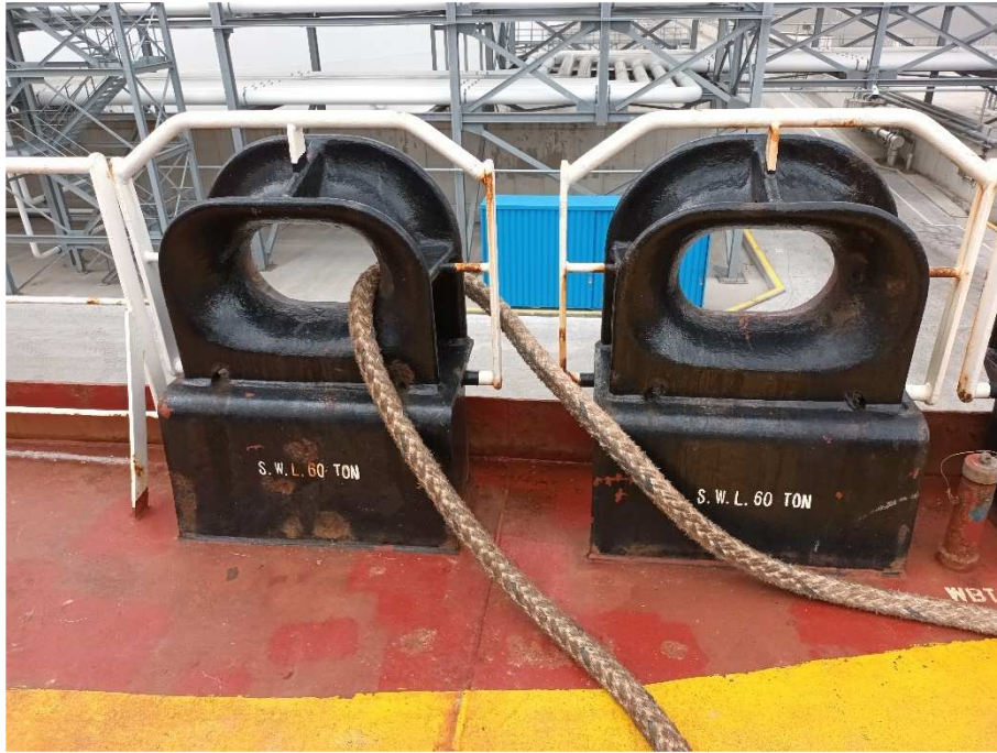
Figure 4 - Broken spring line through Panama lead
