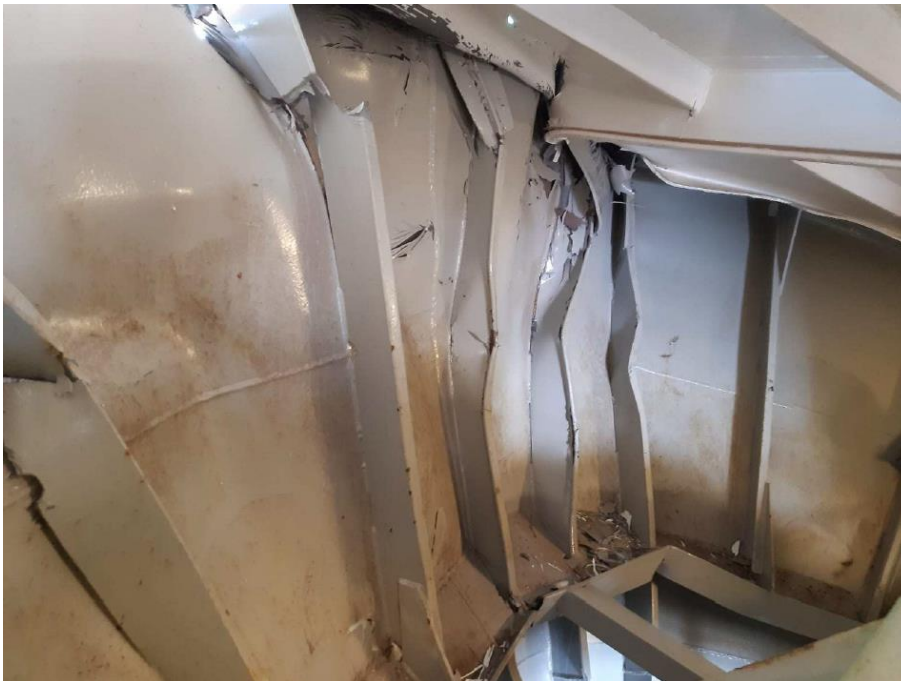
Figure 14 - Damaged stiffened plate structure at the stem of fv Z.575-HEIN SENIOR
