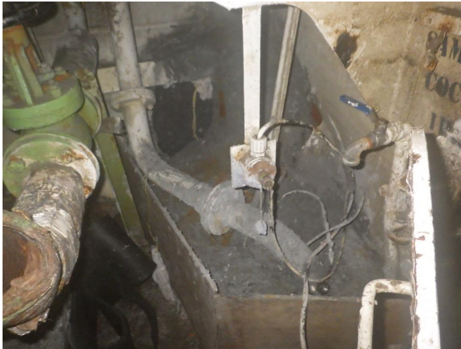
Figure 7 - Water ingress from FW tank into the pump room
