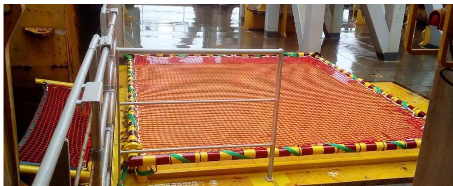
Figure 13 – Sliding gate and permanent railing
