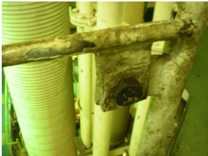
Figure 8 - Bolt used as spigot for section of railing
