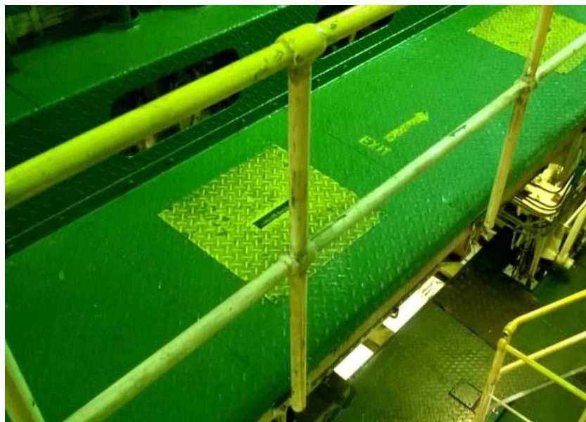
Figure 7 - Typical section of fixed railing in engine room of the mts “EUPEN”
