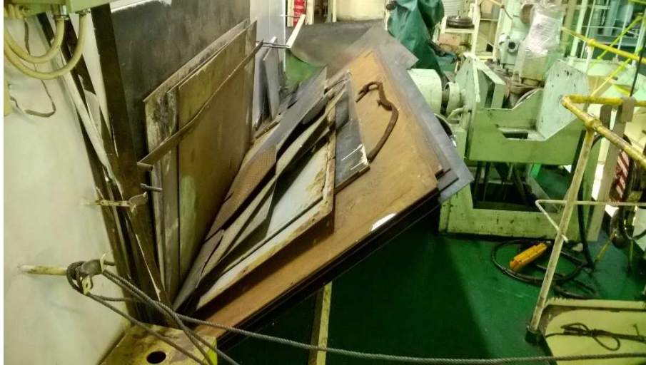
Figure 2 - Fallen metal plates after securing nuts had been removed
